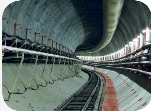
Transporteur en console Belt conveyor on bracket on wall
